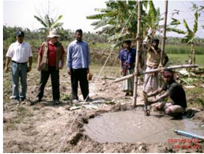
Bild 3: Brunnenbau für Trinkwasser Picture 3: Construction of a well for drinking water
